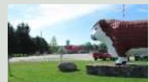
Standpipe in rear, Big Bruce in foreground
