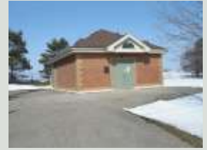
Well No. 1 pumphouse
