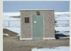
Well No. 2/3 building
