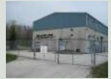
Shallow Lake water treatment building
