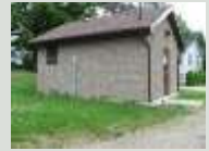
Tara Well No. 2, installed 1960
