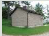
Tara Well No. 4, installed 2006
