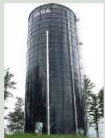
Tara Standpipe, constructed 2010
