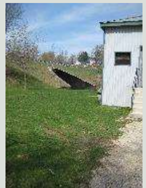
Pumphouse for well
