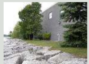
Wiarion Water Treatment Building
