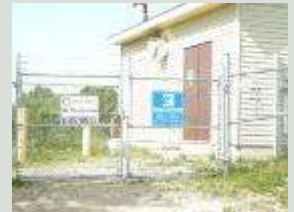
Foreman Water Works
