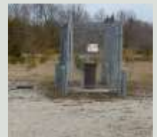
Walkerton Drinking Water System Well No. 9 installed 2001
