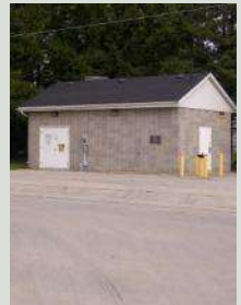
Well No. 1B
