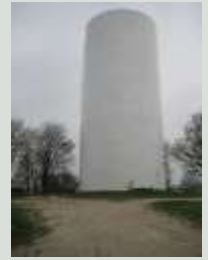
Markdale Standpipe constructed 1986
