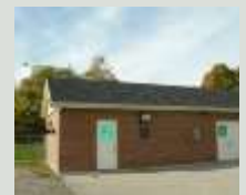
Markdale Well No.3/4 Pump house
