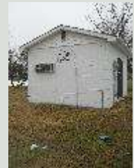
Tiverton Dent Well Building
