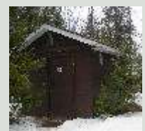
Tiverton Well Building
